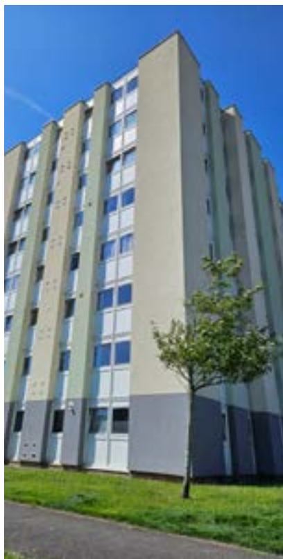
Bruton House 8 storeys (18.16 metres)
